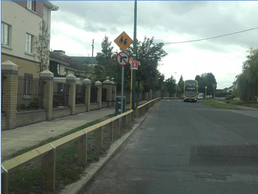
Knee high rails installed on Beneavin Road
